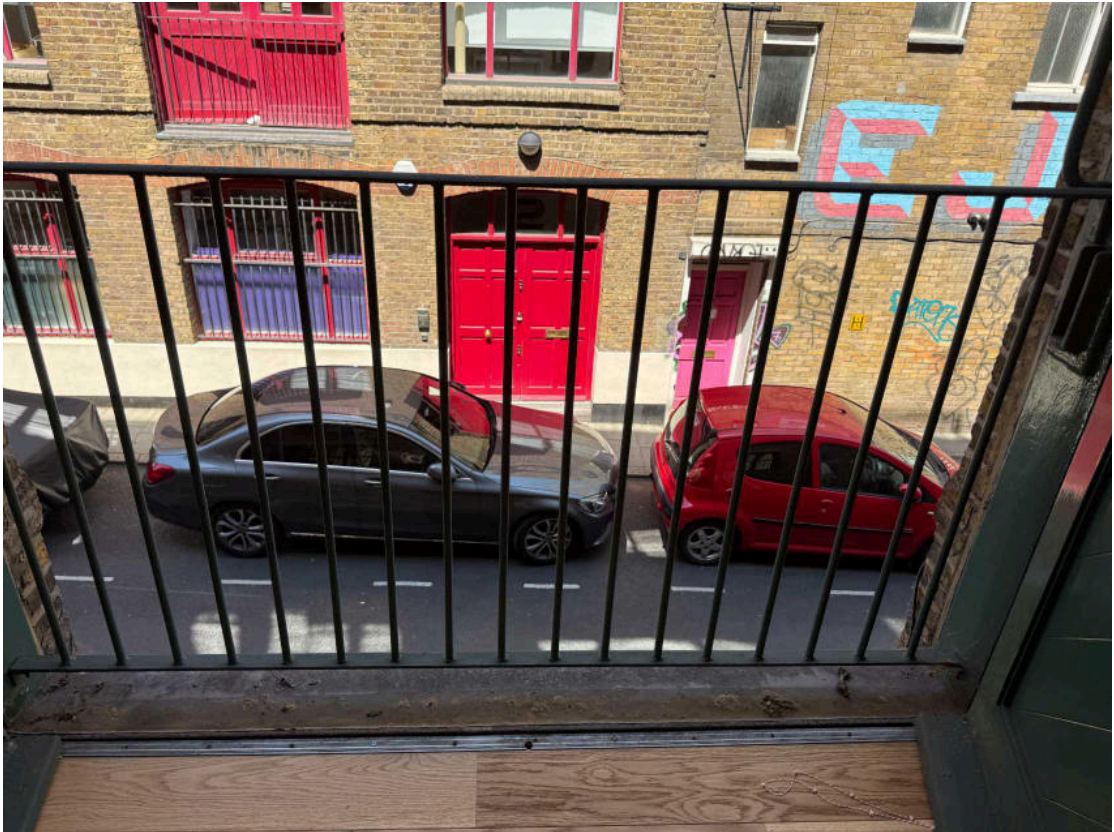
Metal railing to the Juliet balcony
