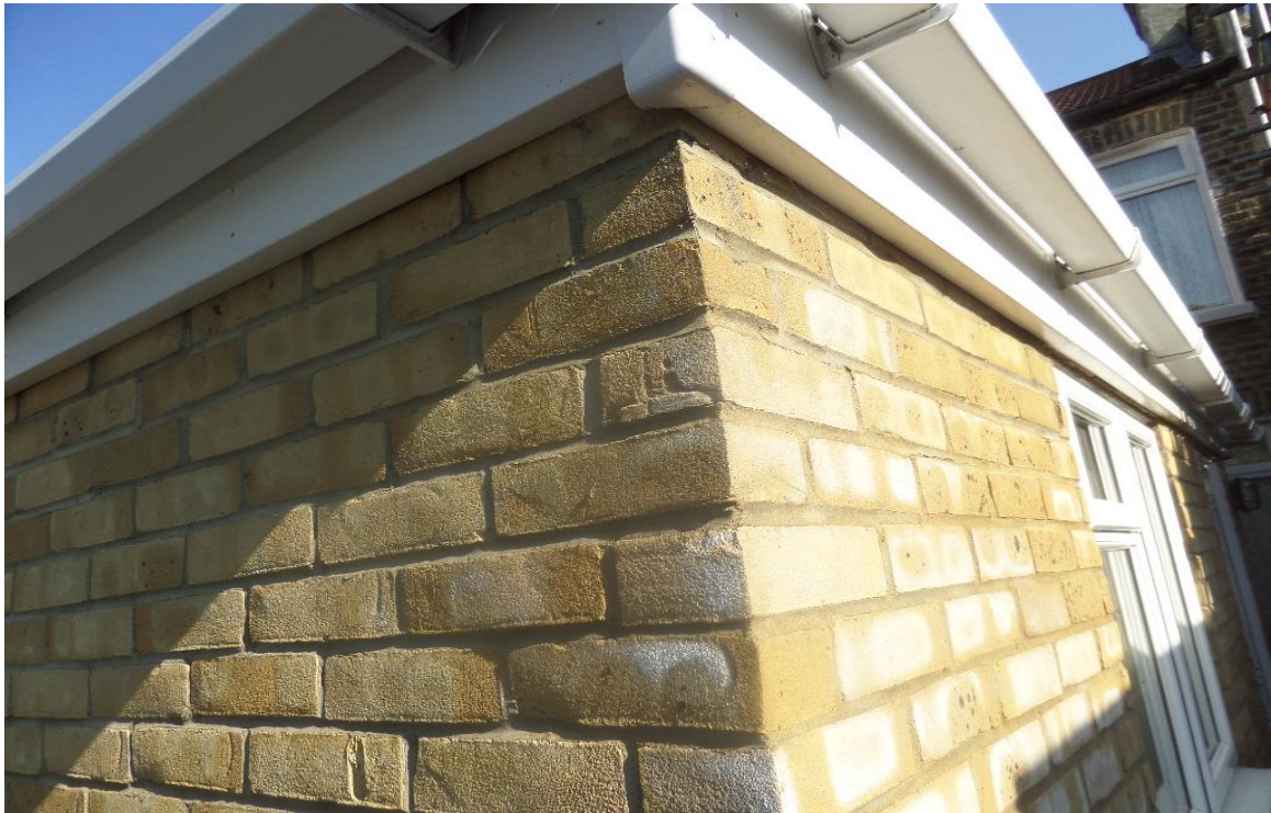
Rear extension wall adjacent to the work site.
