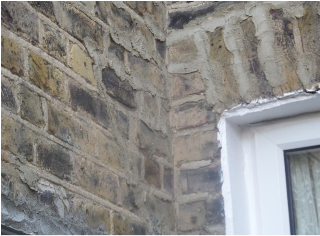
External wall (left-hand side).
