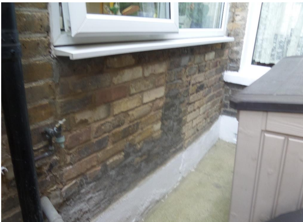
External wall (left-hand side).
