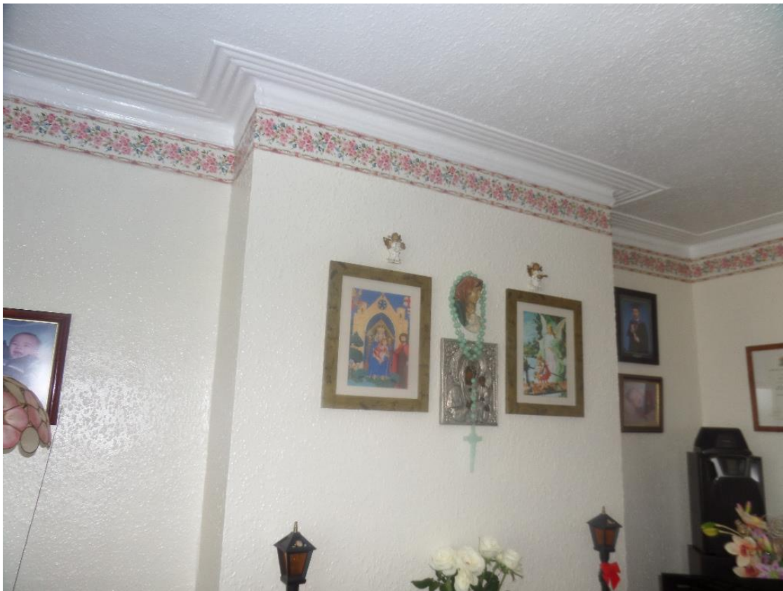
Reception room wall adjacent to the work site.
