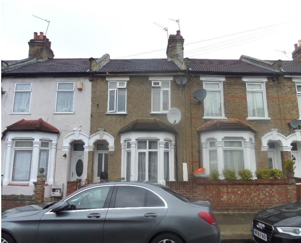
External wall (front).
